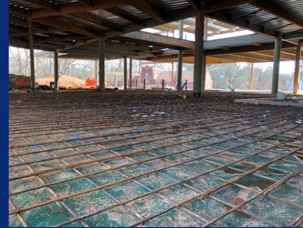
Reinforcing install ongoing ahead of concrete pour in polished area
